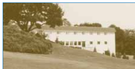
New Caron Hospital is dedicated.
